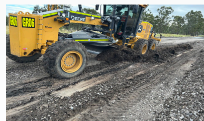
Leveling the soft subgrade prior to laying geogrid.
