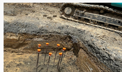
Clean excavated trench through Tensar InterAx.
