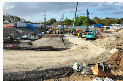
No deep rutting was observed on the stabilised platform.
