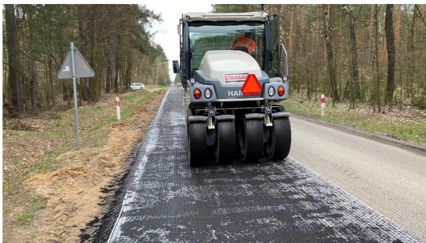
Figure 7: PTR compaction process conducted after product installation and brushing processes
