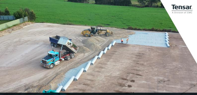
Laying and compacting the first layer of mechanically stabilised layer on the subgrade
