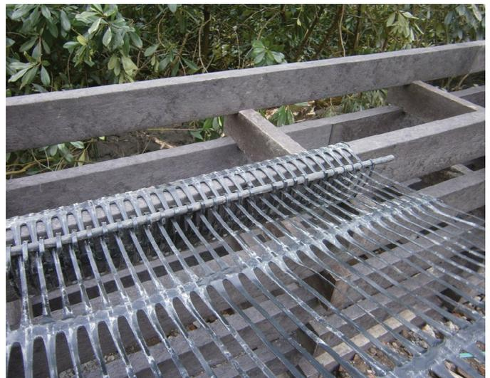
*Tensar bodkin connectors offer high efficiency connection between crib stretcher and Tensar geogrid.*
