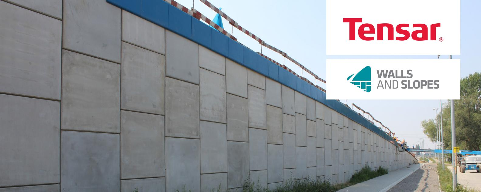
The geogrid reinforced soil system, with fully connected concrete panel facing.
