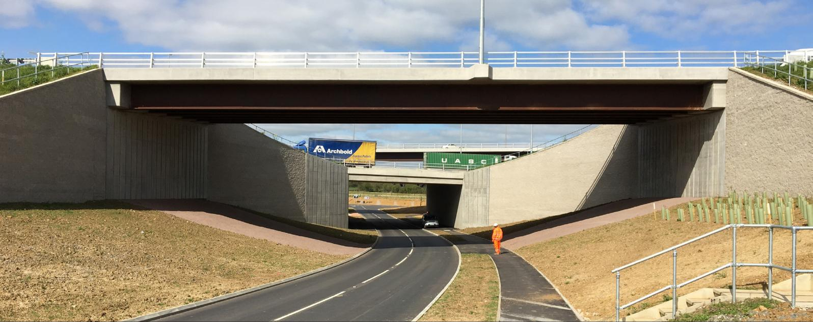
TensarTech TW3 was used to build wing walls and retaining walls for three structures.
