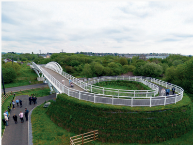
Tensar's TensarTech GreenSlope system easily accommodated the curved geometry and provided a natural looking embankment.
