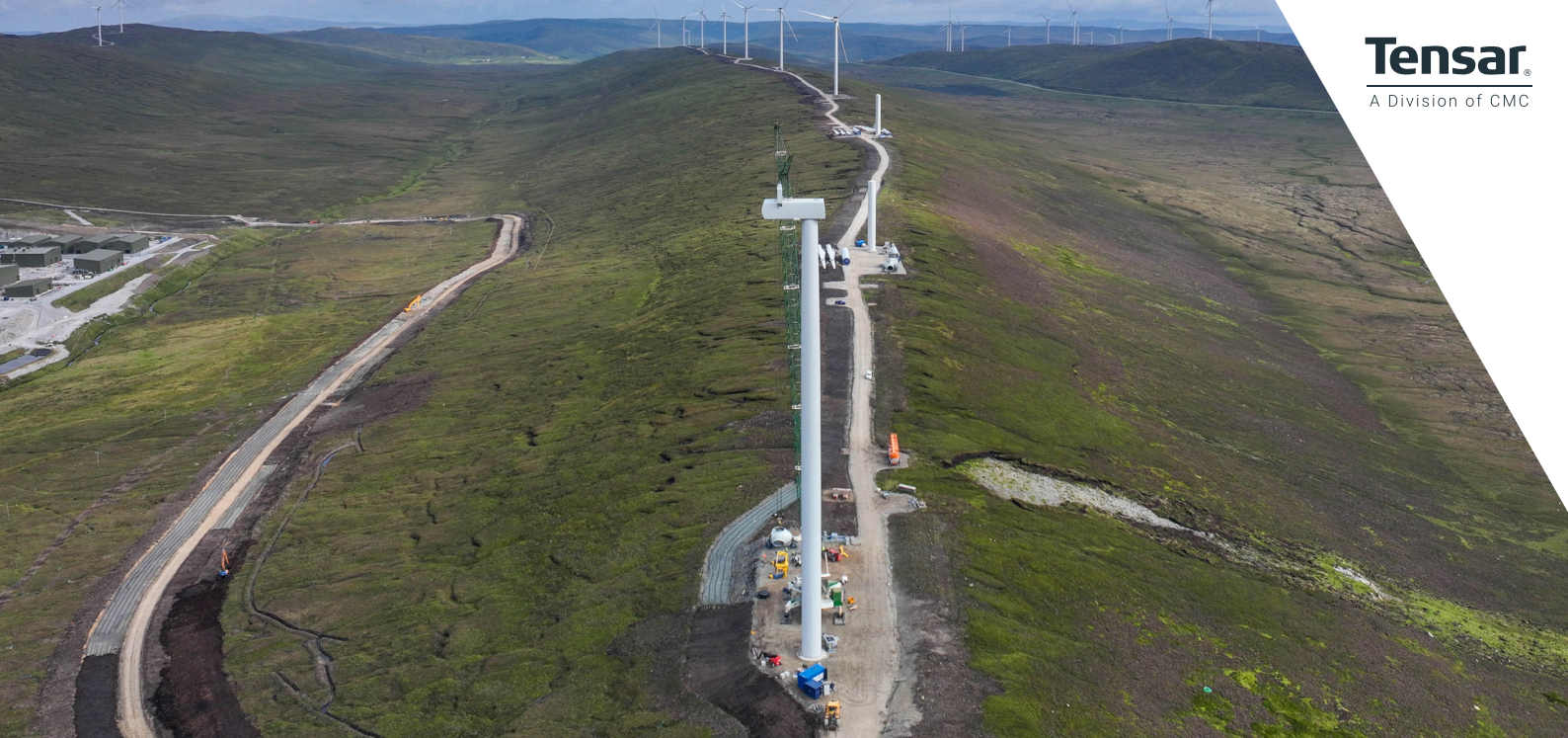
Final turbine installation - the last of 103, with access tracks constructed as 'floating roads' stabilised with Tensar geogrid
