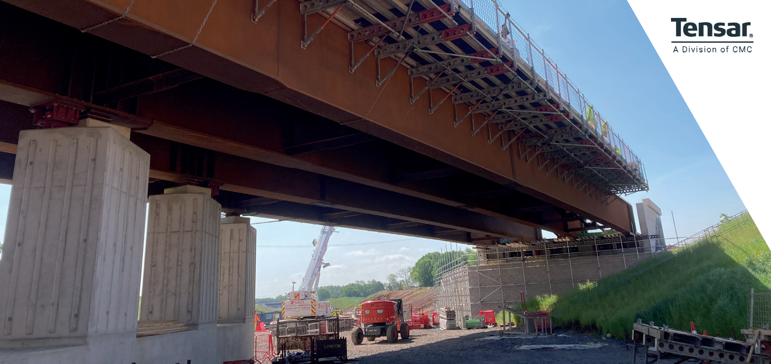
TensorTech TW3 abutments support semi-integral bankseats carrying vertical and lateral bridge deck loading.
