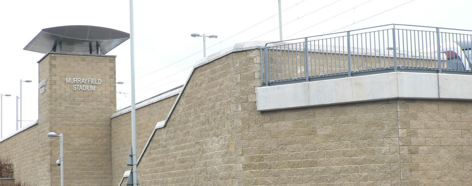
TensorTech® TW3 modular block retaining walls form complex structures at the Murrayfield Stadium tram stop.
