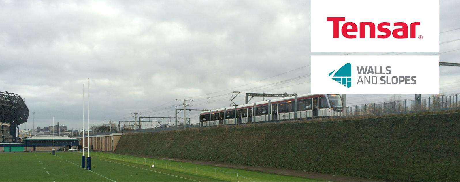
TensarTech® GreenSlope was used to create natural vegetated slopes alongside rugby pitches at Murrayfield Stadium tram stop.
