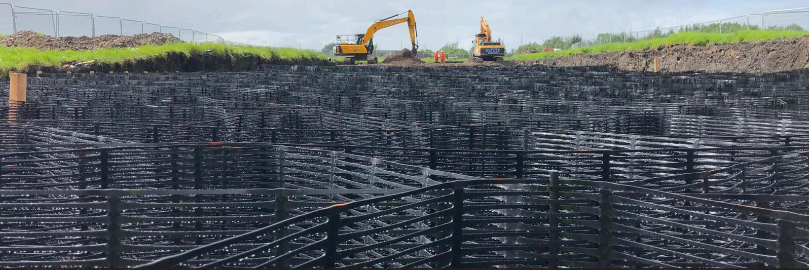
Up to 300m<sup>2</sup> of Stratum was installed by hand per day, regardless of the weather, with cells filled with compacted, recycled granular fill.
