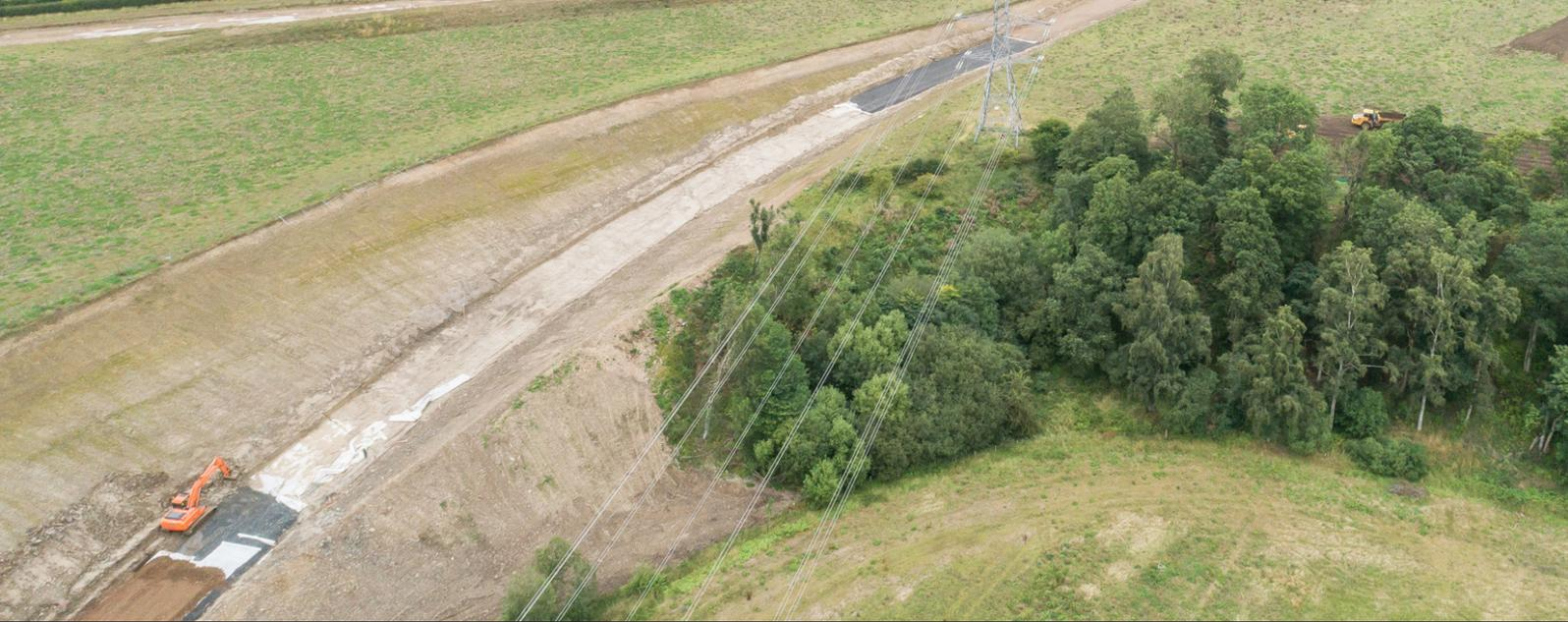
At Bertha Cut, the new link road passes through an area of very weak soils with groundwater level higher than the road.
