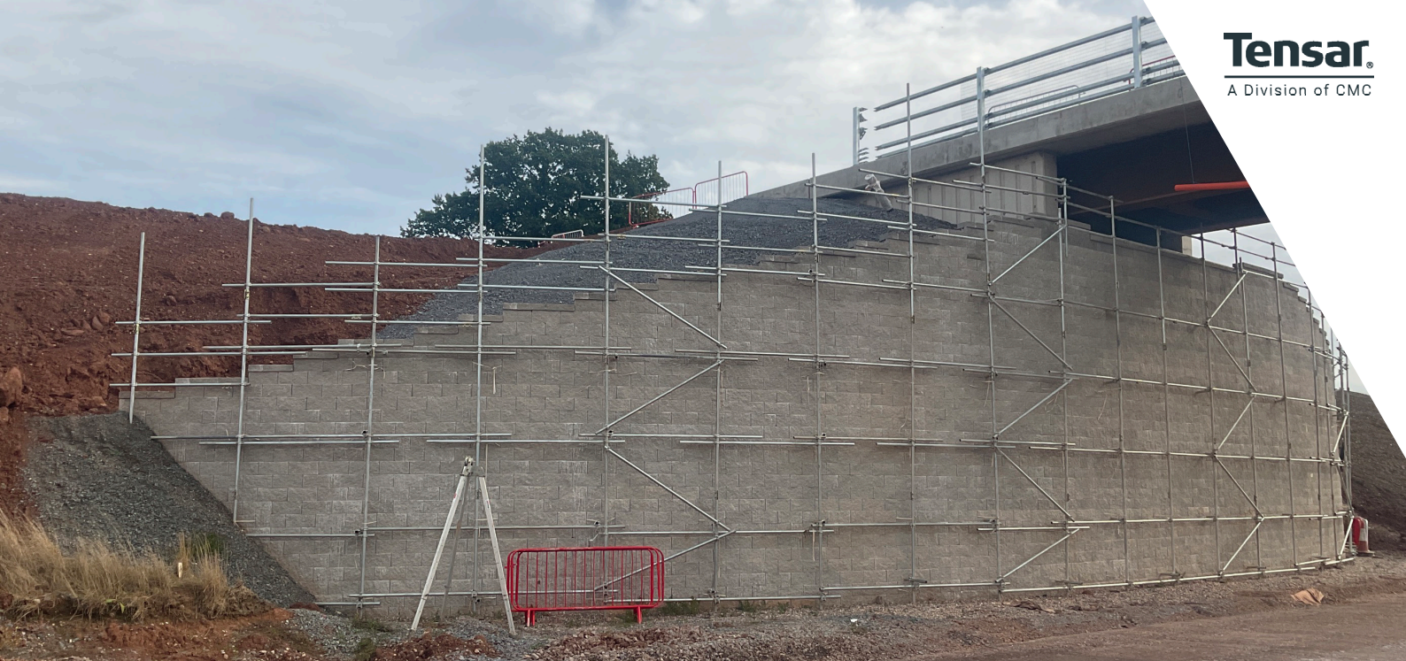
TensorTech TW3 bridge abutment and wing wall nearing completion. Lightweight scaffold is for safety working at height only.
