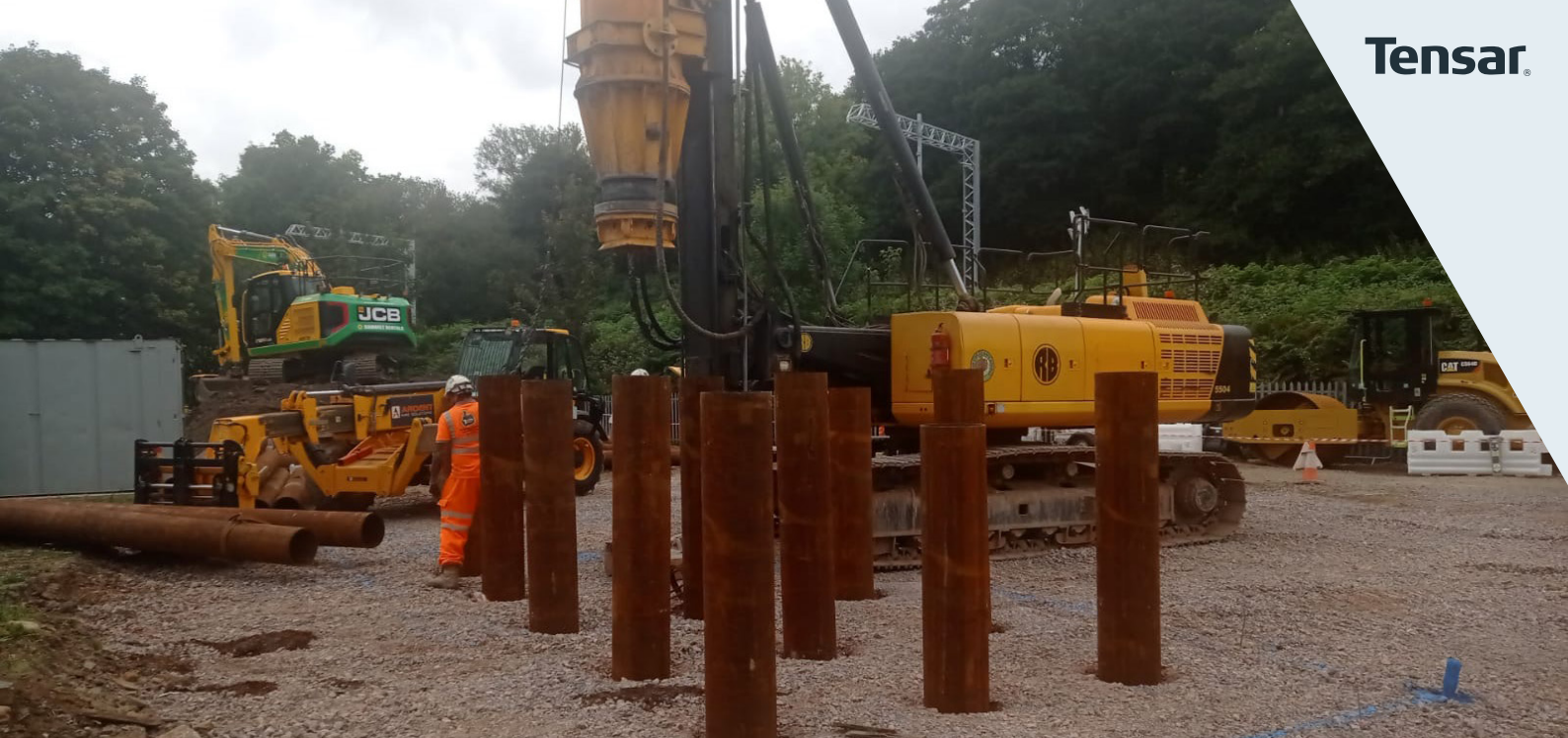
Rig safely operating on a Tensor mechanically stabilised working platform
