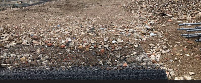
Incorporating stabilising geogrid in the piling mat's granular material meant it could be 33% thinner, without a loss in bearing capacity or load transfer efficiency.
