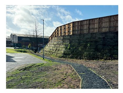
"Tensar's system allowed poor quality, site-won material to be utilised in the construction of this noise-bund, and the flexibility of Tensar's systems allowed strict spatial constraints to be achieved"
