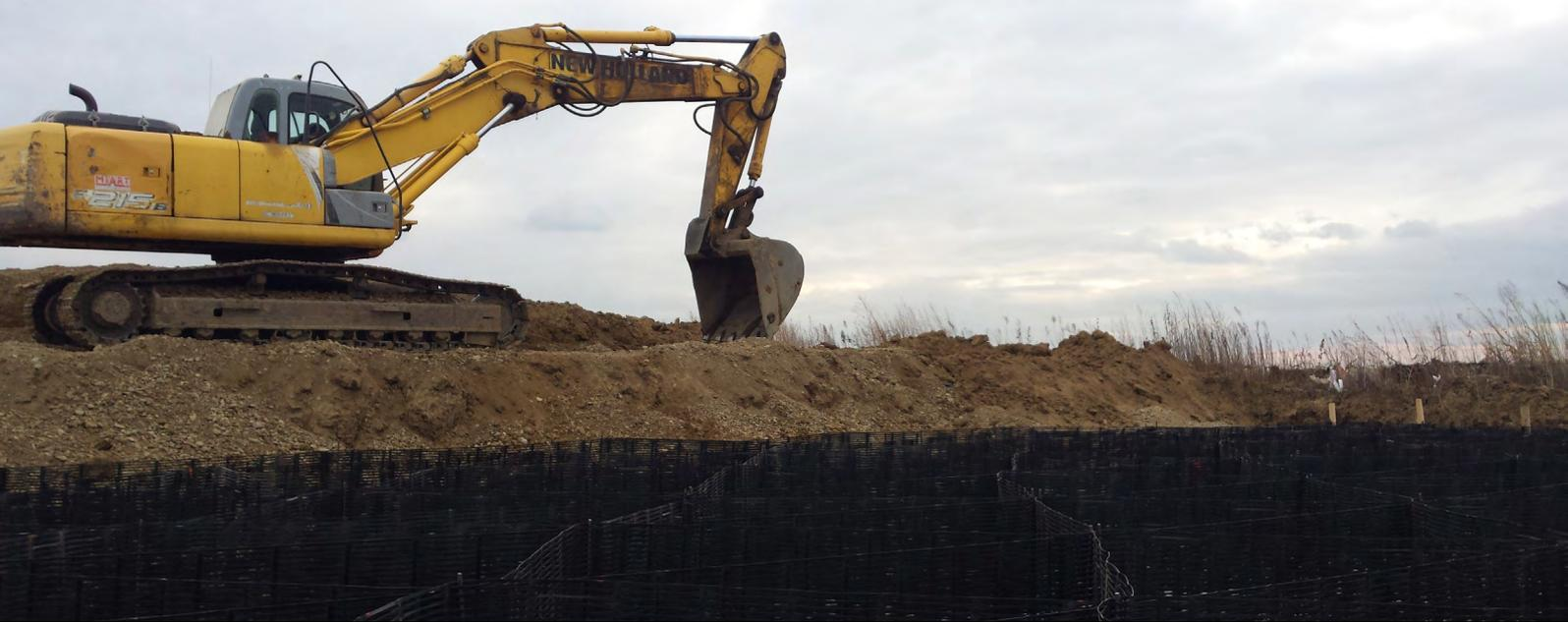
The cells were filled with granular fill, which was compacted to create a stiff raft foundation providing improved stability, increased bearing capacity and minimising overall settlement.
