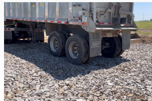
Trafficking truck during installation of well graded granular fill
