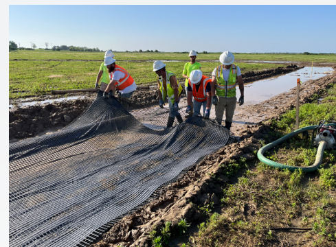
Difficult installation of biaxial geogrid with poorly laminated fabric requiring extra hands to install
