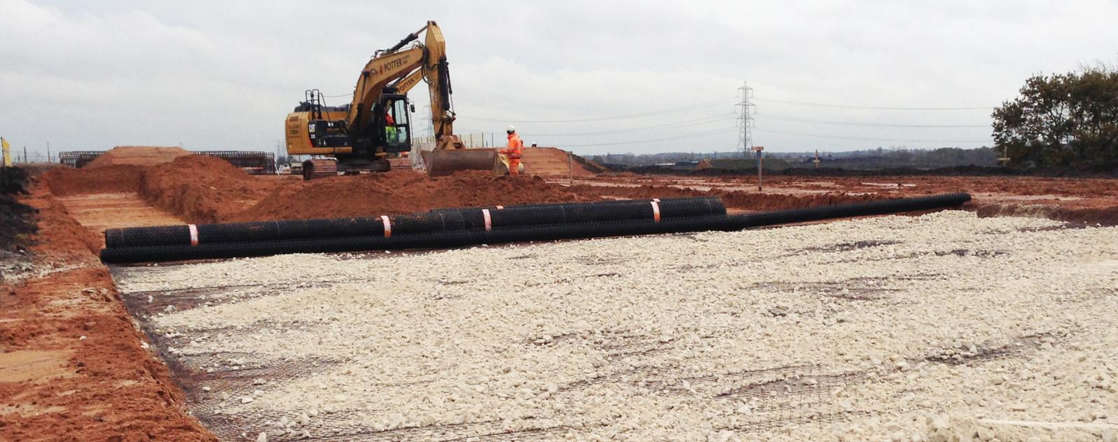
TriAx mechanically stabilised the road subgrade, resulting in a thinner pavement but improved road performance.
