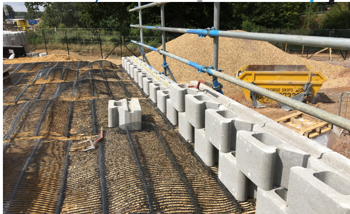
Grafham Road Bridge and B1514 Junction
