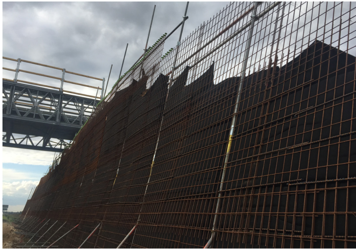
Swavesey Junction improvements
