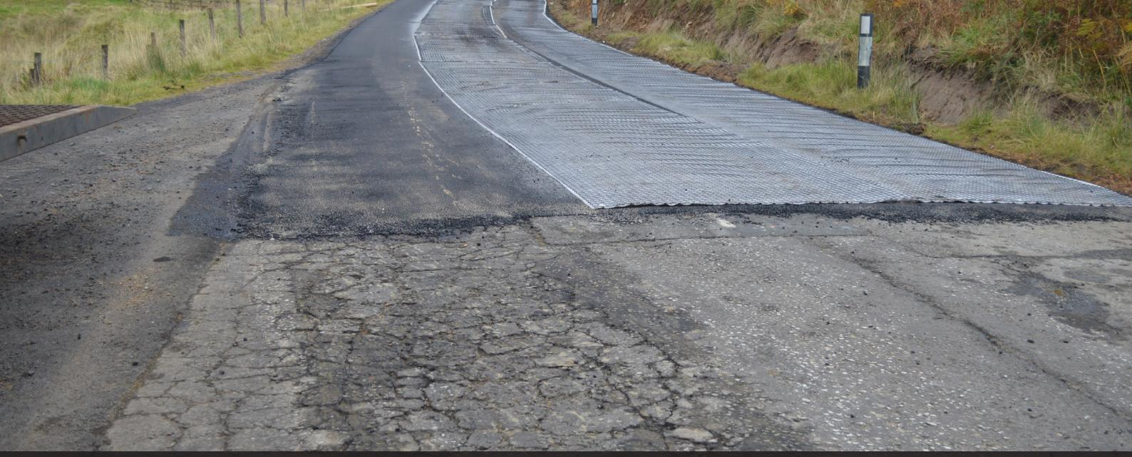
Tensar AX5-GN asphalt interlayer installed onto a 20mm regulating layer.
