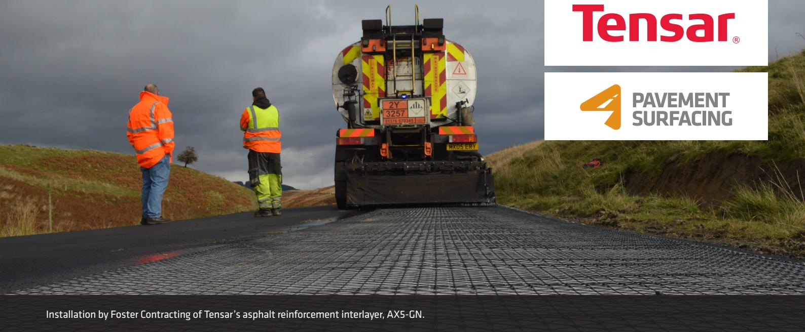
Installation by Foster Contracting of Tensar's asphalt reinforcement interlayer, AX5-GN.
