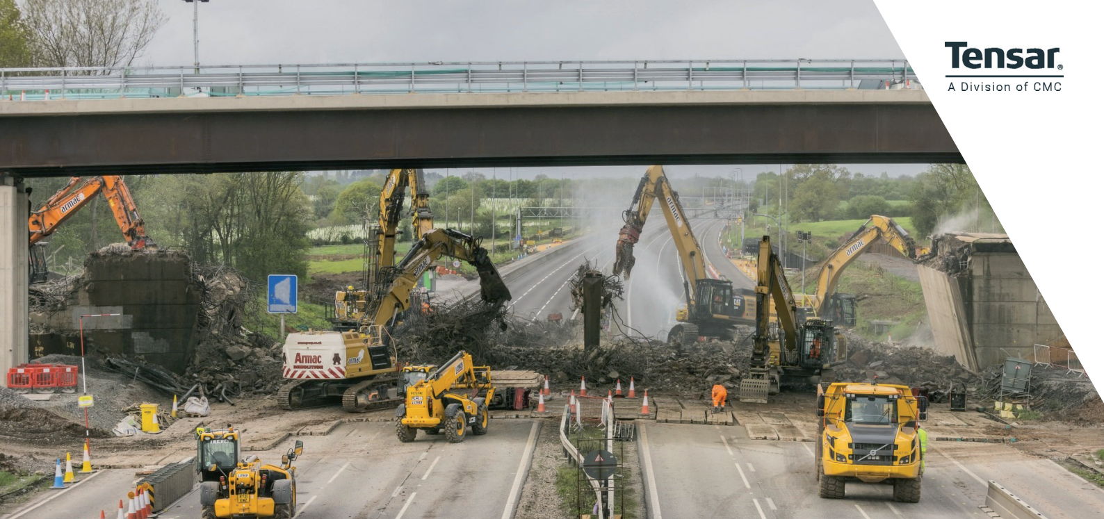
Demolition of the old bridge after opening of the new adjacent overbridge (photo credit: Highways England)
