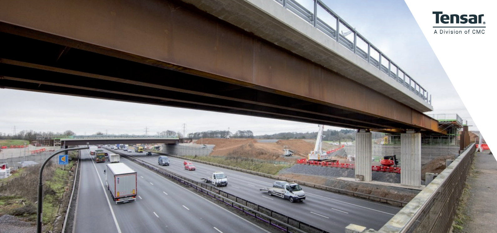
3-span overbridge supported on TensarTech TW3 bridge abutments over the M42 motorway (photo credit: Highways England)
