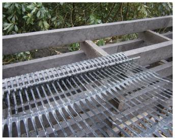
Tensar bodkin connectors offer high efficiency connection between crib stretcher and Tensar geogrid.
