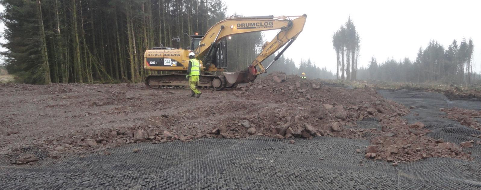
TriAx geogrid was incorporated into the aggregate used for the wind farm access roads and working platforms, cutting material use dramatically.
