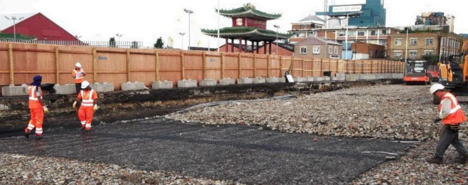
Tensor's working platform design, with TriAx geogrid incorporated in recycled granular material.
