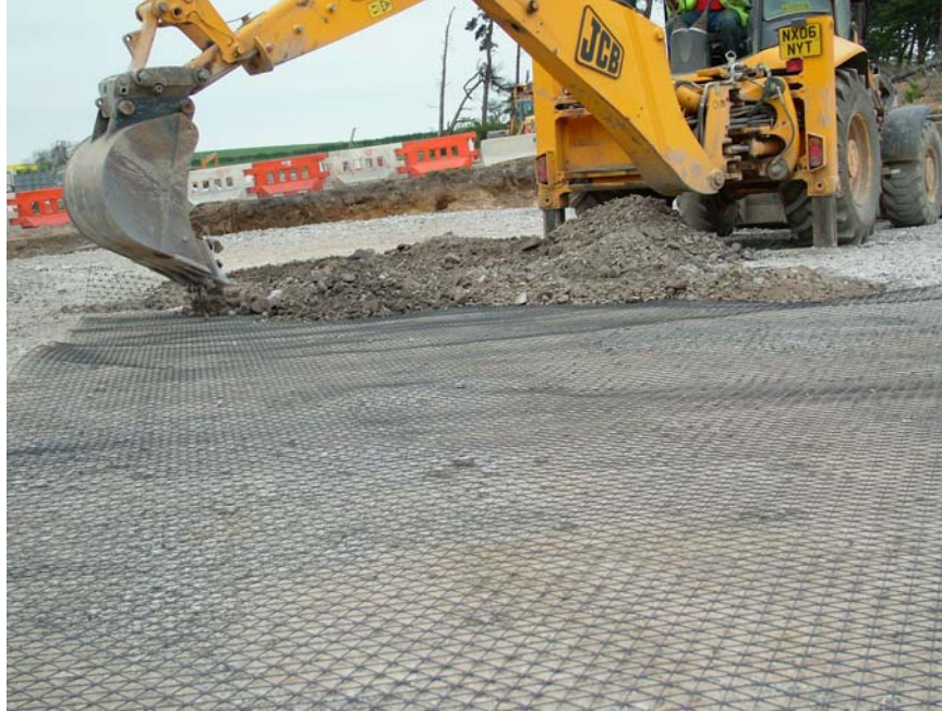
Tensar TriAx™ during installation
