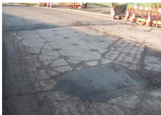
Crack and seat before regulating course
